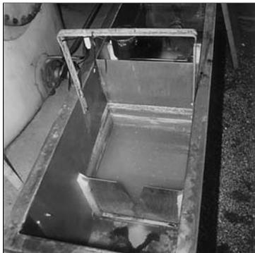
*Measuring box supplied for wastewater outlet at dairy. With the little flow that is measured it is best to use a prefabricated measuring box where the 90° weir is mounted directly on the measuring box.*
